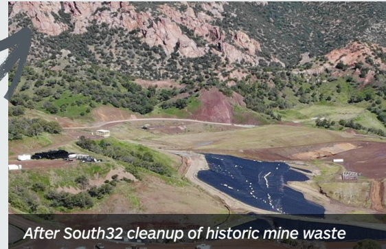
Before South32 cleanup of historic mine waste
